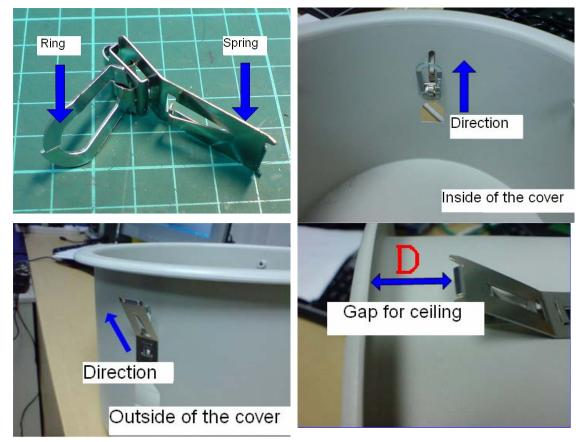
3. Push this outer cover into the ceiling. Check if the leaf springs are clipped to ceiling tightly.
